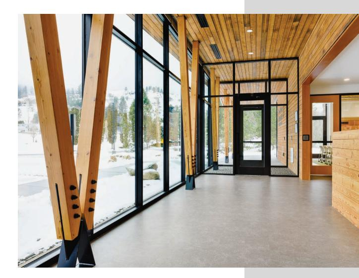
Mass timber building showcases work of the U.S. Forest Service ountering the concept that mass timber is only suited for expensive urban buildings, the U.S. Forest Service (USFS) chose cross-laminated timber (CLT) and glue-laminated timber (glulam) to build a new supervisor's office for the Nez Perce-Clearwater National Forests. The two-story structure, built in the small town of Kamiah, Idaho, fits seamlessly into its remote, scenic location.
