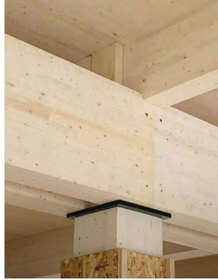
Column connected to CLT beam and girder
