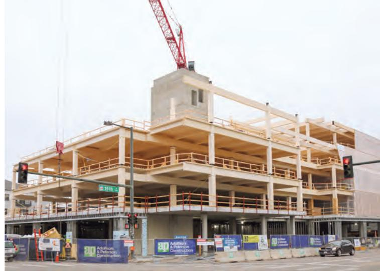
Mass timber reduced construction time by 20%
