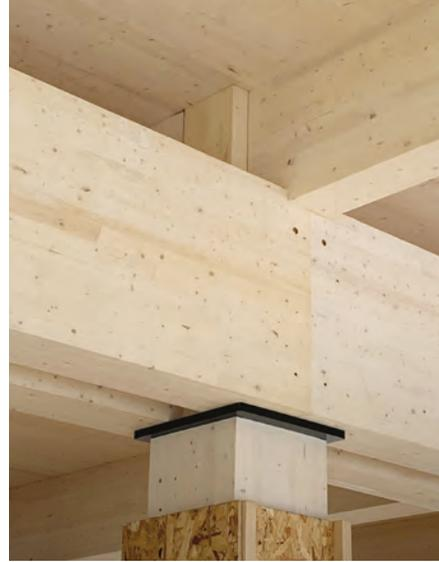
Column connected to CLT beam and girder
