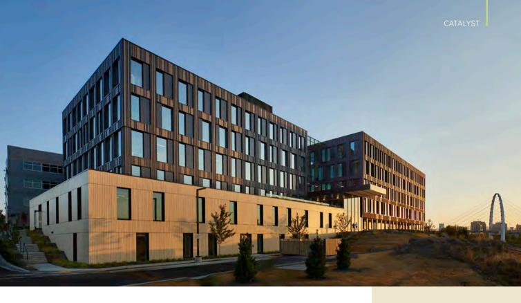
A ptly named for its goal of inspiring new ways to build, Catalyst is the first cross-laminated timber (CLT) office building constructed in Washington state and the first to use panels produced at Katerra's new CLT production facility. It is also designed to Passive House principles and to achieve zero-carbon
