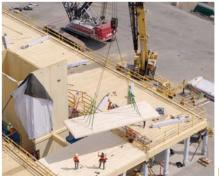
Catalyst is the first CLT office building in Washington State, and the first to use CLT panels produced at the new Katerra facility in the Spokane Valley. The use of CLT means the building will have a smaller carbon footprint than comparable buildings built with steel and concrete.
