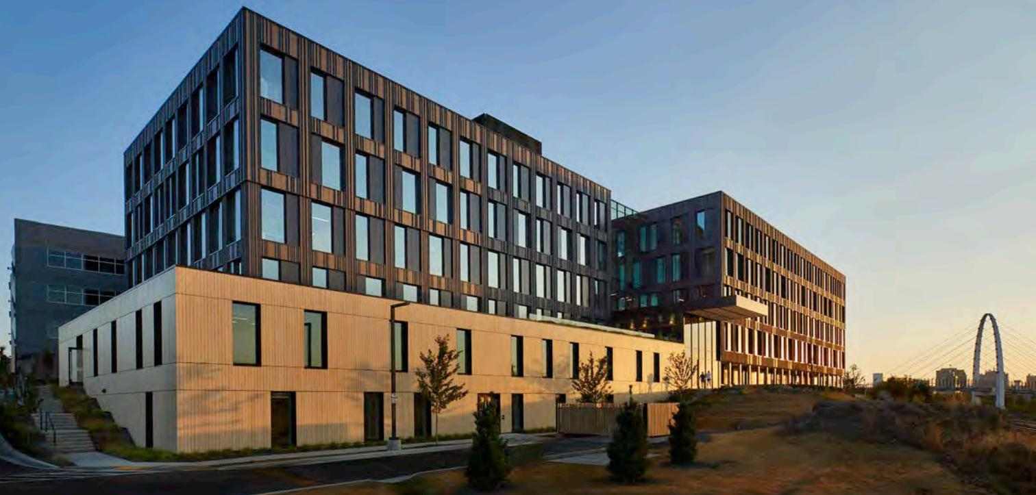
**A**ptly named for its goal of inspiring new ways to build, Catalyst is the first cross-laminated timber (CLT) office building constructed in Washington state and the first to use panels produced at Katerra's new CLT production facility. It is also designed to Passive House principles and to achieve zero-carbon and zero-energy certification from the International Living Future Institute (ILFI), making it a leading example of sustainable building design.
