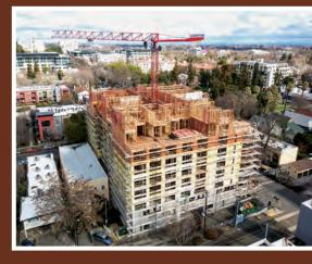
For years, the International Building Code (IBC) allowed light wood-frame buildings up to five stories for residential occupancies (six for office) over a single-level podium. The 2015 IBC evolved to recognize multi-level podiums, which had been permitted in the Seattle Building Code for some time. Across the country, designers began maximizing the value of their midrise projects with 5-over-2 configurations; however, 5-over-2 still wasn't sufficient to make the investment in 1430 Q pencil out.
