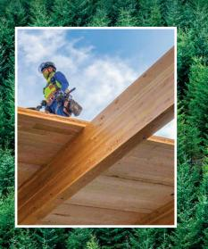
Silva added, "Our ability to go with a 3-ply CLT panel was driven in part by our decision to run four inches of structural concrete topping on top of the slab. When we played with the bay spacings, we learned that the 10-foot span worked with a 3-ply panel if the panel was E-rated. This optimized the fiber within the structural frame while still meeting the layout needs of the classrooms, labs and other spaces within the building."
