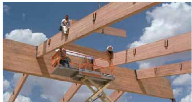
*Pre-engineered glulam beams were methodically assembled on-site for the Gunter Primary School in Gunter, Texas. At nearly 60,000 square feet, wood-frame construction for the school cost just under \$100/square foot. Credit: APA – The Engineered Wood Association*
