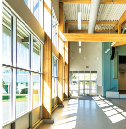
At Morris E. Ford Middle School, exposed wood columns are raised off the floor to protect against moisture.
