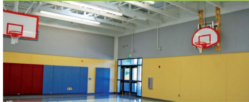
At Shining Mount Elementary School, corridor wall finishes include MDF, vinyl and gypsum. MDF is also used on the lower section of gymnasium walls.
