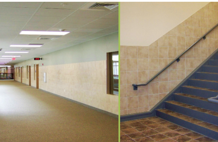
At El Dorado High School, hard tile covers the lower 6 feet of corridor walls and stairwells.
