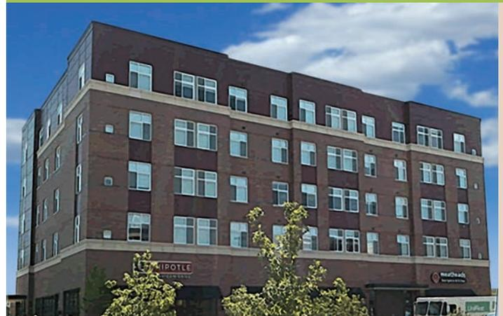
The first phase of this mixed-use development (Flats on Main, a 28-unit apartment complex) featured wood for the interior partitions and the floor and roof framing systems, but the engineer chose heavy 12-gauge steel studs for the walls. Because the contractor overwhelmingly favored the ease of construction of the wood partitions, the second phase of the project (Flats on Osage) eliminated the steel studs and used wood framing throughout.
