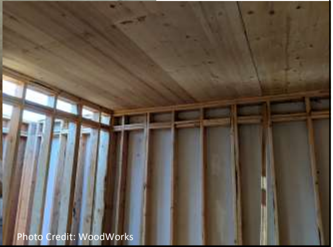
Cheney Park Apartments CLT floor on Panelized Light Frame Walls
