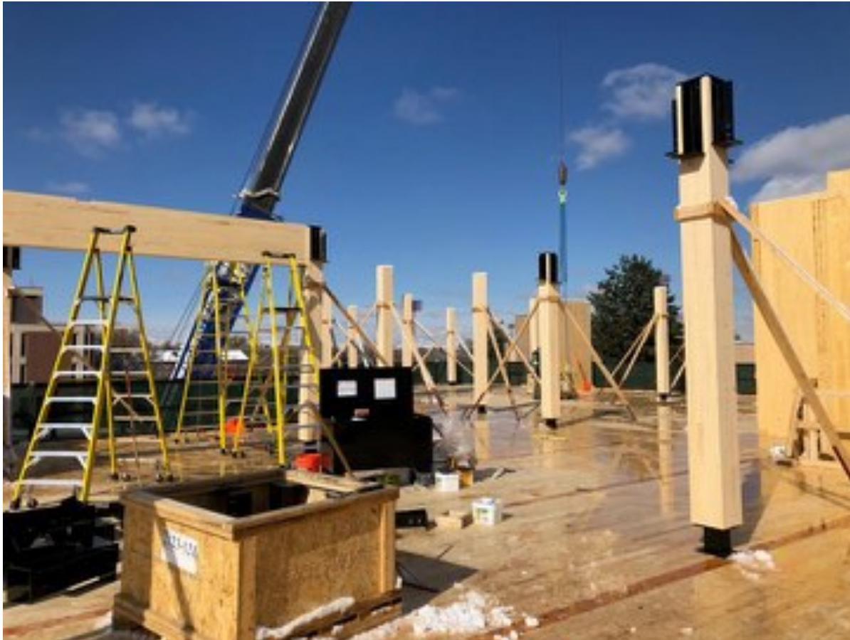
GLU-LAM BEAMS AND COLUMNS (NOTE SNOW IN FOREGROUND AND COLUMN BASE CONNECTION)
