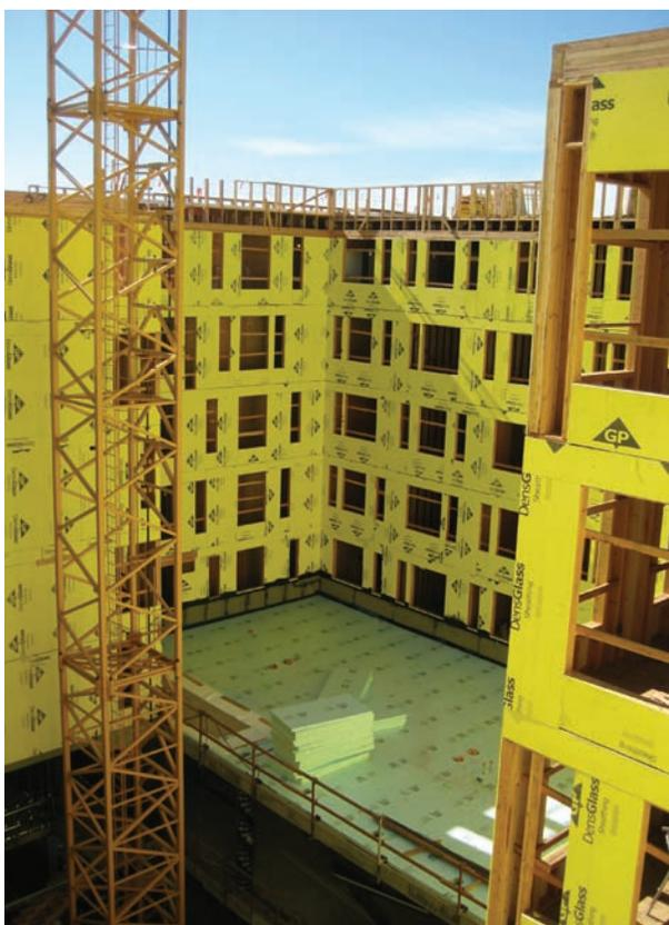
SSA also made recommendations for structural to reduce floor vibration. They recommended that the live load deflection of the floor assembly between residential units should achieve a max L/480; the code only requires L/360. They also recommended that plywood sheathing be placed only on the outer side (not the inner side) of double stud walls, since air space between the layers of mass on each side of the studs is critical for achieving the specified acoustical performance.
