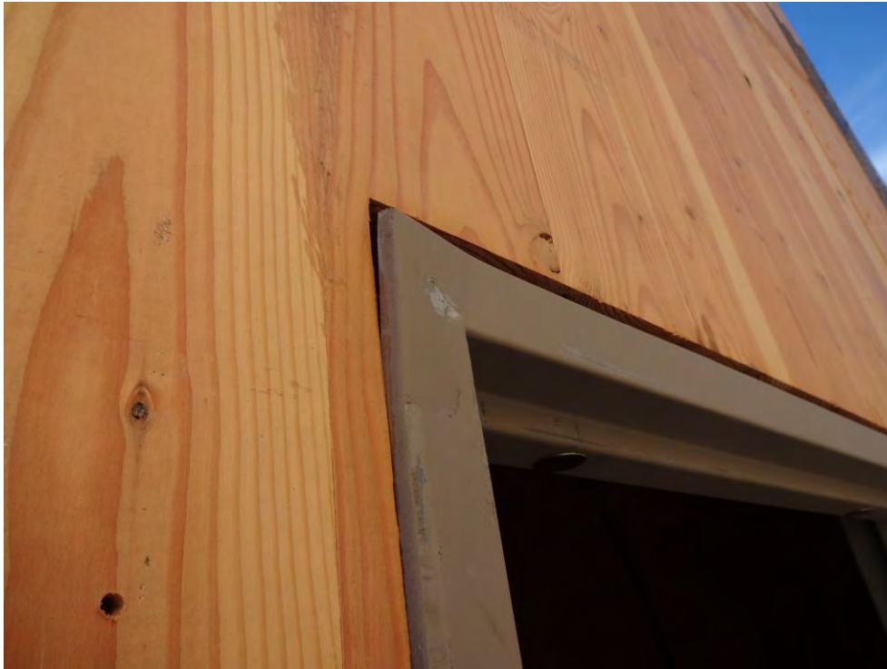
(a) Door Frame Inelastic Deformation.
