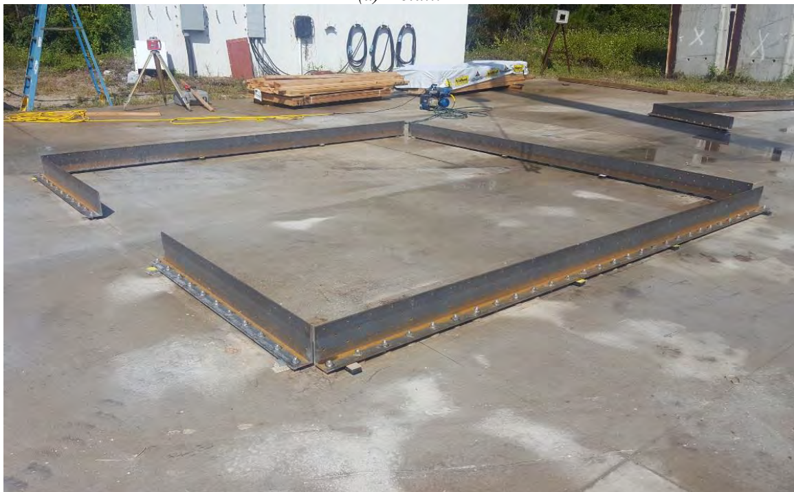
(b) Angle Placement Prior to Panel Install.
