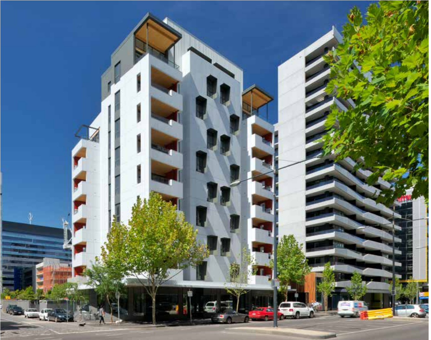
Project Name: Forté Photo credit: Lend Lease Architecture by: Lend Lease
