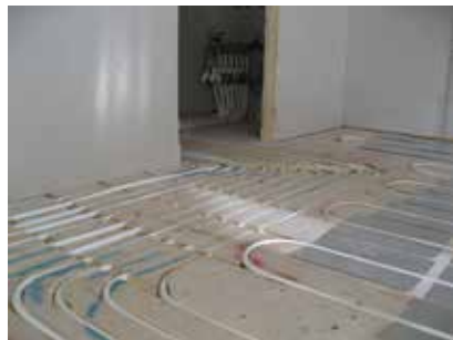
On-site milling for hydronic heating pipes at Limnologen Photo credit: Martinsons Byggsystem
