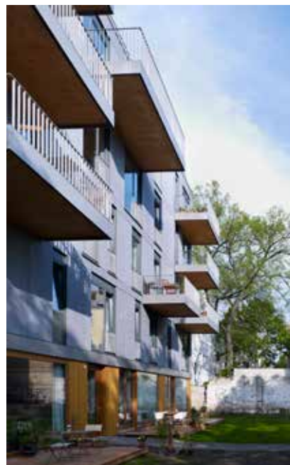
Exposed timber on underside of balconies at 3XGRÜN Architecture by: Atelier PK, Roedig Schop Architekten and Rozynski Sturm Photo credit: Stefan Mueller
