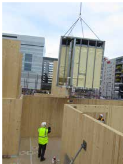
Installation of prefabricated bathroom pod at Forté. Photo credit: Lend Lease
