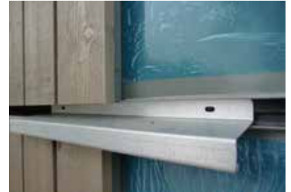
Holz8 exterior wood façade with metal flashing between each storey prevents the spread of fire Photo credit: Huber & Sohn
