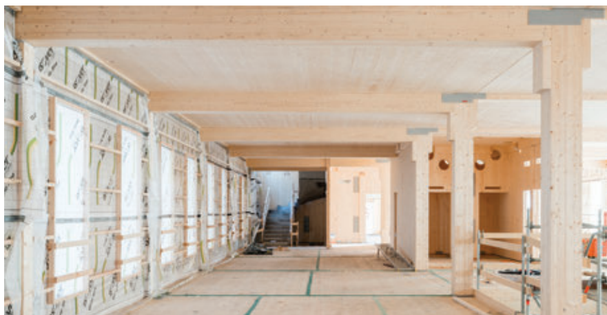
▲ Figure 2.6.4. GLT columns and beams seen during construction on a level in the low-rise podium. © Martinsons | Jonas Westling
