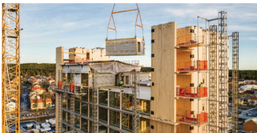
▲ Figure 2.6.5. A prefabricated CLT module, which will form one of the hotel rooms, is lifted into place. © Martinsons | Jonas Westling
