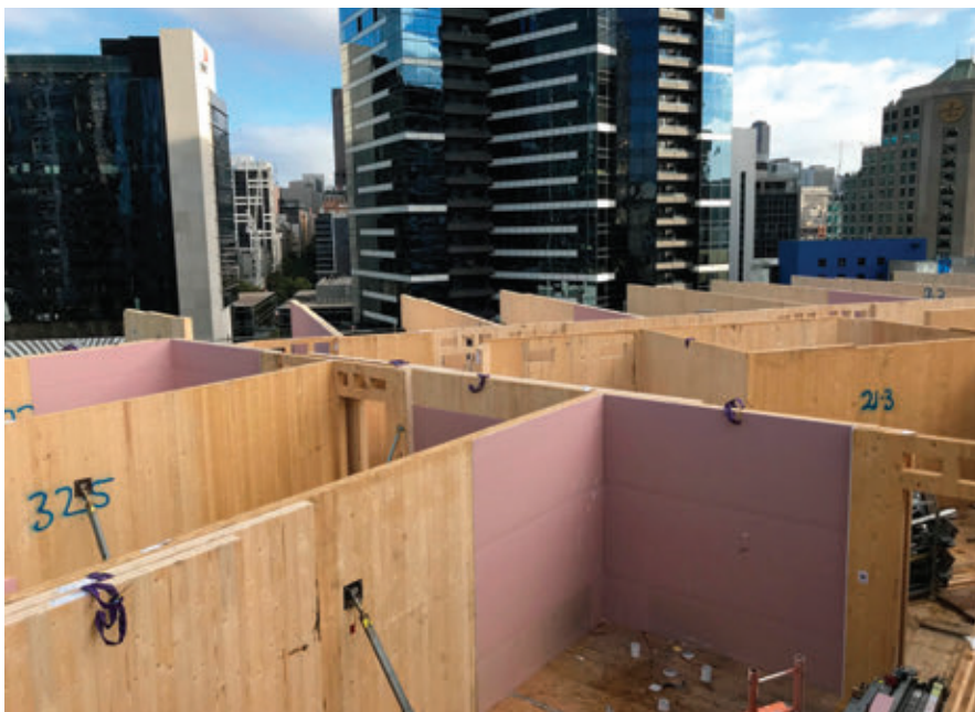
▲ Figure 2.1.8: CLT panels arrived on-site pre-cut with openings for MEP services, easing the installation process. © Robert De Brincat
