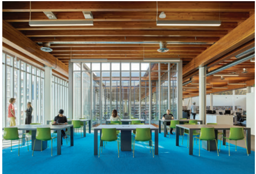
▲ Figure 2.3.2: The interior of Billie Jean King Library showcases the community-centric layout. The long spans are achieved by glulam beams sitting on brackets on either side of concrete-filled steel columns. © Benny Chan | Fotoworks
