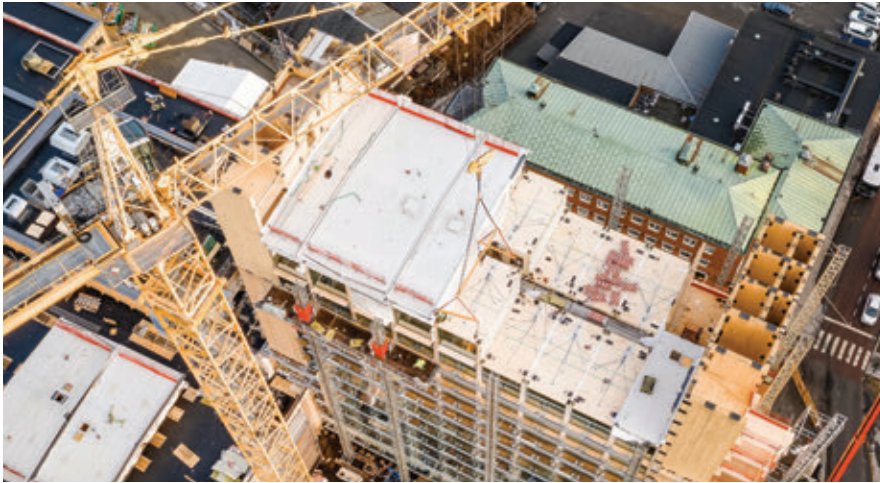
▲ Figure 2.6.22. The installation of the pre-assembled modules for each floor started at the interior CLT core and worked outward, with each module stacking directly on top of the module below. © Martinsons | Jonas Westling
