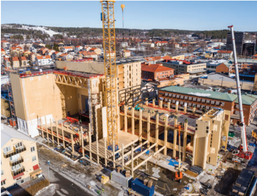
▲ Figure 2.6.20. The installation of the steel box truss on level 5, surrounded by construction on the lower floors. © Martinsons / Jonas Westling
