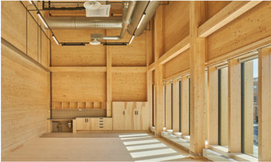
▲ Figure 2.6.17. In many public areas of the podium, high ceilings made hanging MEP ducts and pipes an unobtrusive proposition. © Åke Eson Lindman
