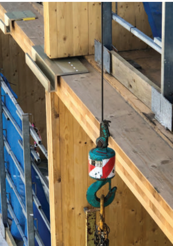
▲ Figure 2.1.9: A crawling crane was used for raising façade elements into place, which could then be bracketed to the CLT floor panels. © Bates Smart
