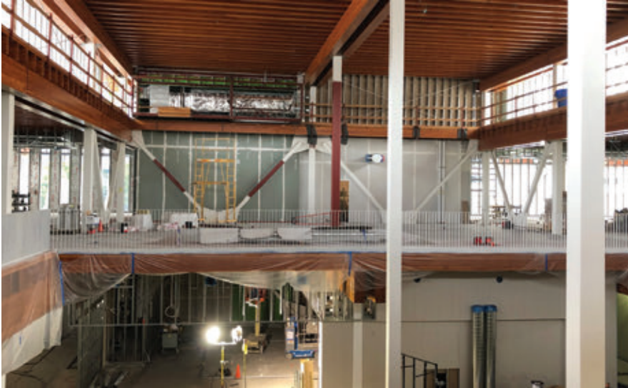
▲ Figure 2.3.6: Corner connection detail, showing the concrete-filled steel columns, glulam girders and joists, and plywood decking. © SOM
