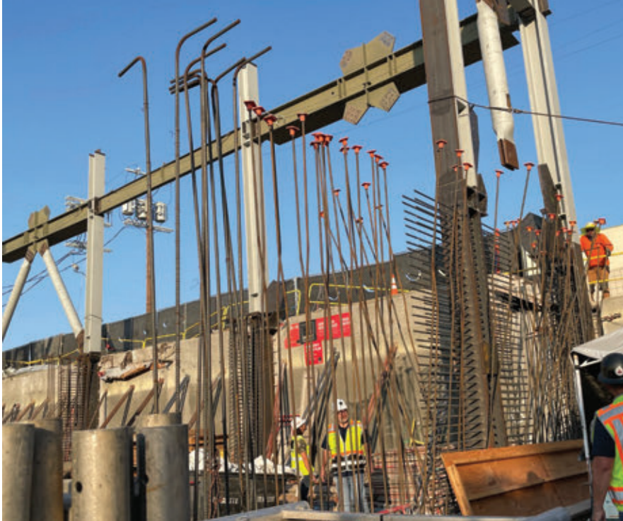
▲ Figure 2.2.4: Steel columns (W14x) are placed atop existing 14-inch (366-mm)-diameter concrete columns, then fitted with the steel wide-flange perimeter frame. Round HSS braces are on view at upper right and center left. © LEVER Architecture
