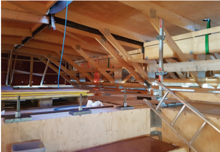
▲ Figure 2.5.10. Underneath the temporary roof, the tops of the LVL walls with post-tensioning bars and anchor plates visible at center-left. © Mika Keskisalo
