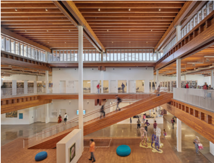
▲ Figure 2.3.8: An interior photo of Billie Jean King Library, highlighting the significant presence of exposed timber and the clerestory window surrounding the atrium. © Benny Chan | Fotoworks
