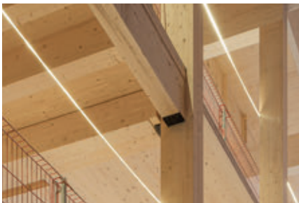
▲ Figure 2.6.8. Detail of the column-beam-platform system used on the lower floors. © Martinsons I Jonas Westling
