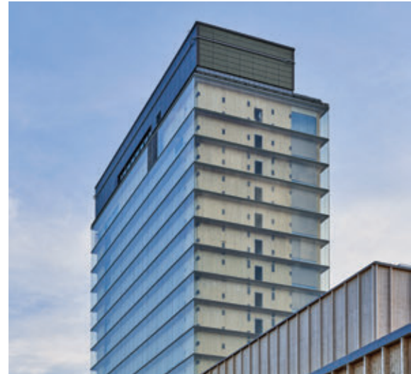
▲ Figure 2.6.18. The building's glass exterior has an air gap, in which sun screens are mounted to the underside of the floor above. © Åke Eson Lindman
