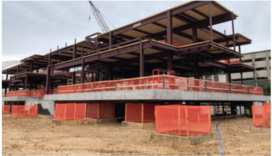
▲ Figure 2.4.4: Construction view of the project, with crawler crane for CLT panel and steel beam and column hoists at center. © Kevin Daly Architects, photo by Iwan Baan
