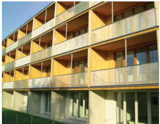
▲ Figure 1.2.6. Spöttlgasse, Vienna. The social housing project has five stories; levels 2–5 are constructed of CLT, over a concrete-framed structure on Level 1. © Sozialbau AG | Vienna
