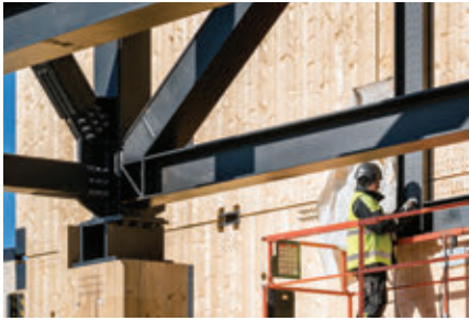
▲ Figure 2.6.6. Detail of the connection between the steel box truss and the GLT column below. © Martinsons I Jonas Westling
