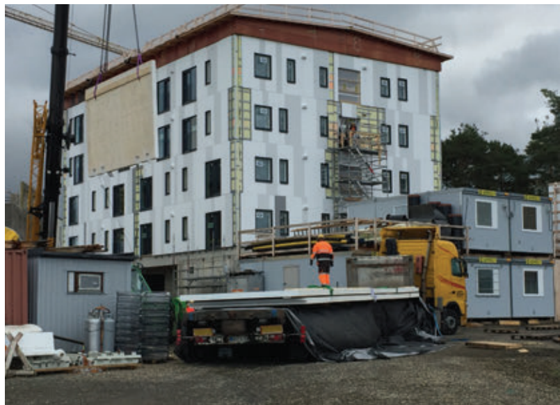
▲ Figure 2.5.9. A panel is lifted from the truck onto the structure. Note the cutouts at bottom for access to tension rods. The roof is temporary, also lifted in and off by crane, for protection of exposed timber and comfort of the workers. © Mika Keskisalo
