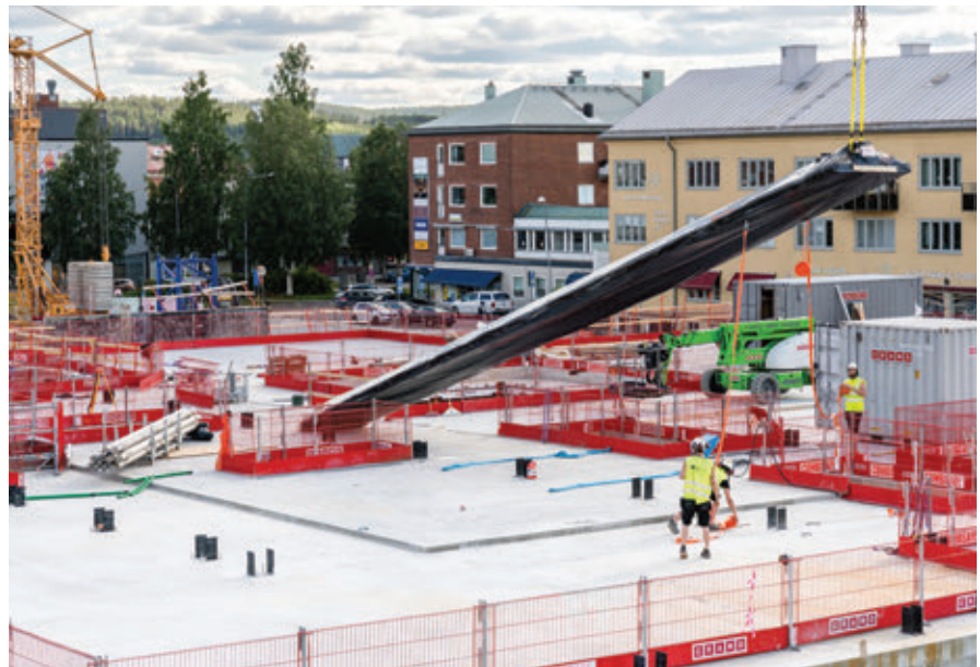
▲ Figure 2.6.19. The CLT wall shown here was kept wrapped until placement and installation of surrounding walls, to protect it from the weather. © Martinsons | Jonas Westling
