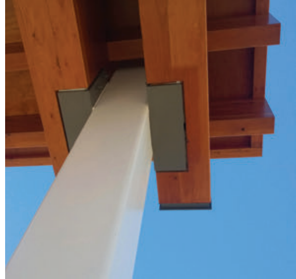
▲ Figure 2.3.5: Corner connection detail, showing the concrete-filled steel columns, glulam girders and joists, and plywood decking. © SOM
