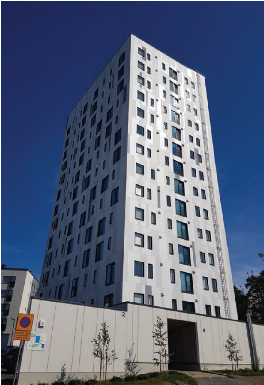
▲ Figure 2.5.1: Overall view of Lighthouse Joensuu, a 14-story student dormitory in Joensuu, Finland. The structure is predominantly LVL and CLT panels, fully encapsulated and stabilized by a system of connected post-tensioning bars. The exterior envelope is an aluminum panel system. © Daniel Safarik
