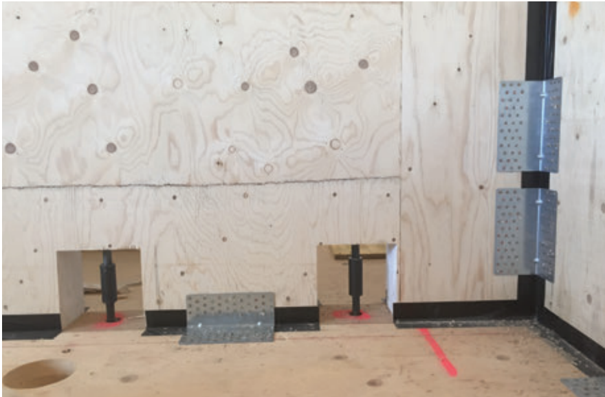
▲ Figure 2.5.7. Wall and floor intersection on the building interior, showing brackets and holes cut for tensioning the rods. © Mika Keskisalo
