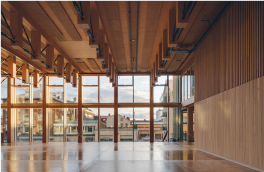
▲ Figure 2.6.16. The automatic sprinkler system is discreetly hung from the underside of the CLT floor panels above the multipurpose room on Level 2. © Martinsons / Jonas Westling
