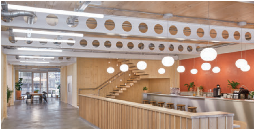
▲ Figure 1.1.6. 6 Orsman Road, completed in London in 2020, utilizes steel beams with mass timber floor plates, allowing exposed timber in the ceiling. © Waugh Thistleton Architects
