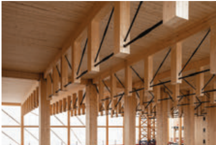
▲ Figure 2.6.7. Detail of the steel-timber truss used for the long spans of the cultural space. © Martinsons I Jonas Westling
