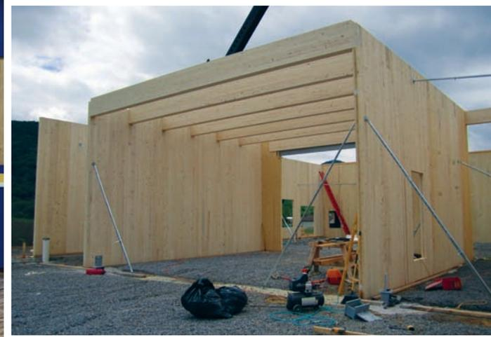
"CLT panel thickness is dependent on span and loads, so when we needed to avoid columns, we just increased the thickness of the CLT floor panels to increase the allowable spans," said Wean. "We did the same for the CLT roof panels, which ranged in thickness from about 5 to 9-9/16 inches, and were nearly 8 feet wide and 40 feet long."
