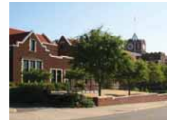
Lincoln High School 100 Years Old – Renovated 2007 AIA & CEFPI Awards Tacoma, WA.
