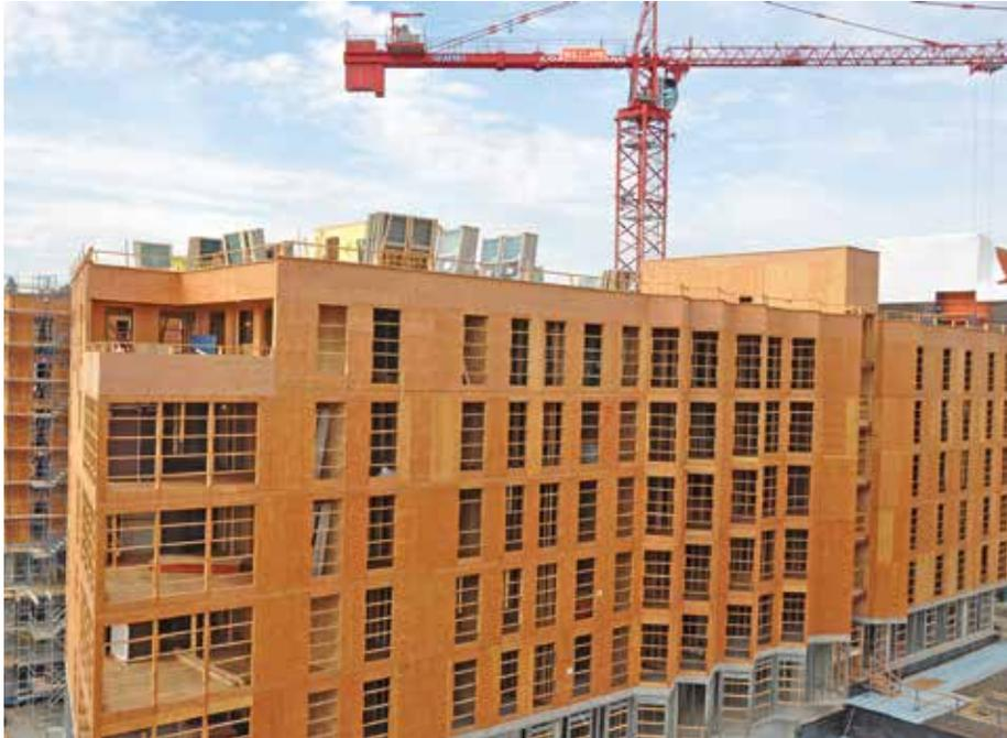
For this project in the Pacific Northwest, plywood sheathing is used as an exterior substrate, onto which the weather-resistant barrier and cladding would be attached.
