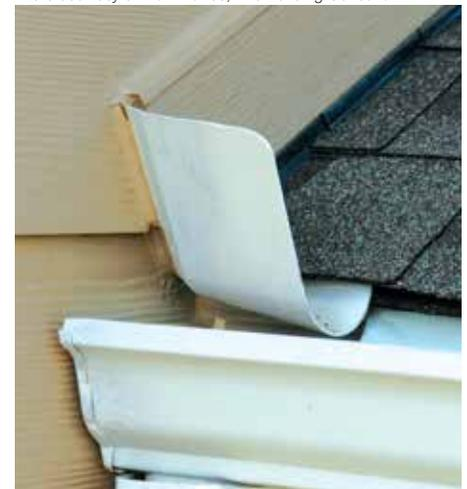
A molded kick-out flashing device efficiently diverts water into the gutter and prevents water intrusion at the roof/wall intersection.
