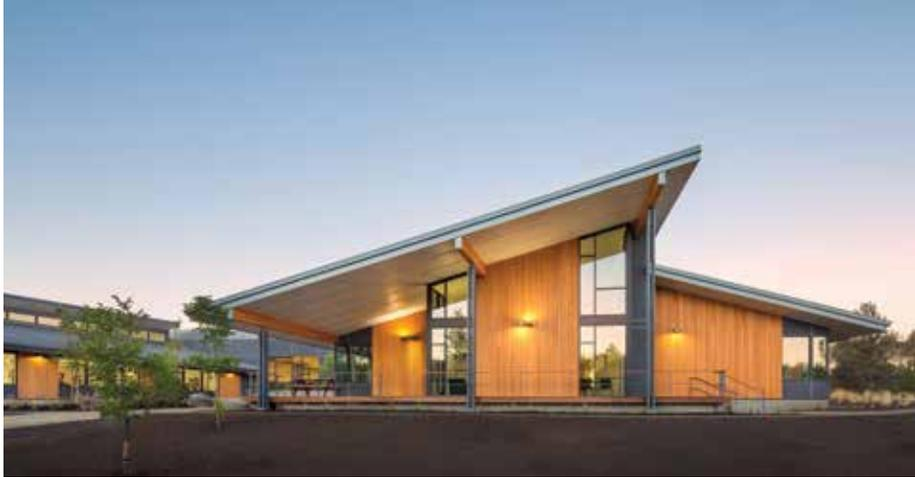
Western red cedar's unique properties make it ideal for weather-resistant applications, including roof shingles, decking, exterior siding, and exterior cladding. At the Cascades Academy of Central Oregon, western red cedar cladding is arranged in vertical sections separated by glazing to reflect the rhythm of scattered junipers and pines.
