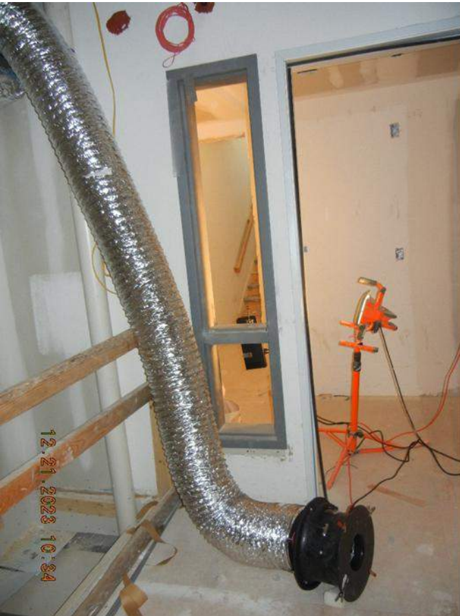
Pressure testing in progress
