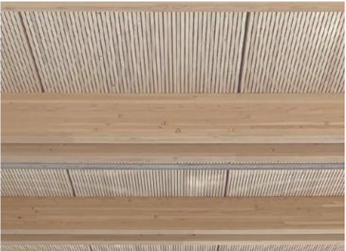
DLT in 2024 Redmond Public Library (Miller Hull project near Bend, OR)
