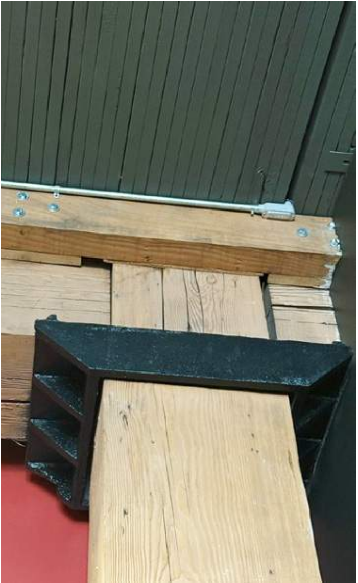
NLT & heavy timber in 1908 Polson Building (Miller Hull's Seattle office)
