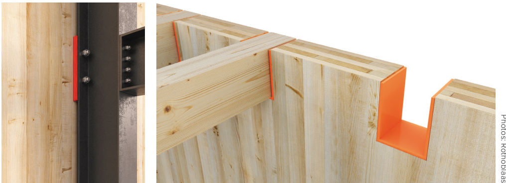
FIGURE 6: Acoustical isolation strips
