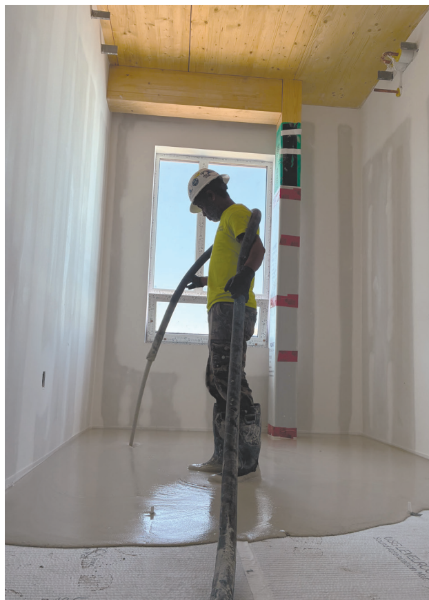
Concrete floor topping
