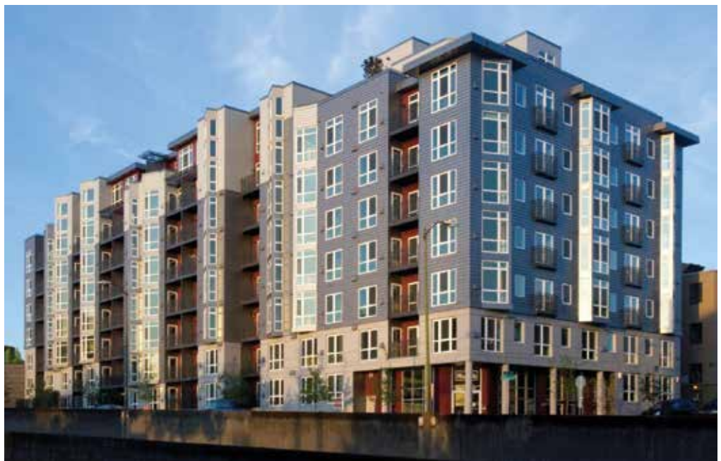
Figure 1. Typical mid-rise five stories of wood framing over the two-story concrete podium.
