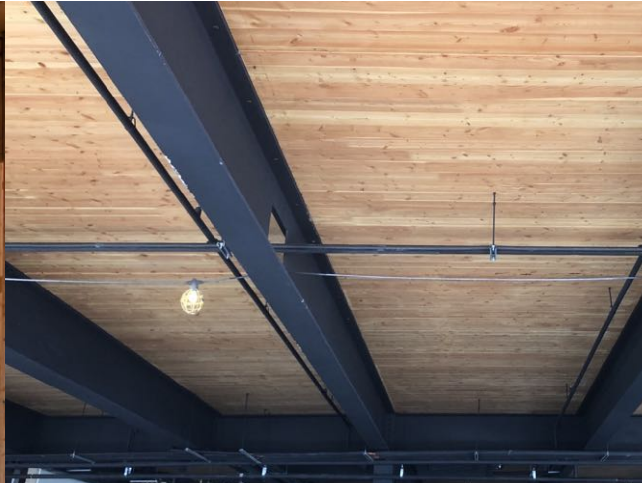
Hybrid: Steel framing
