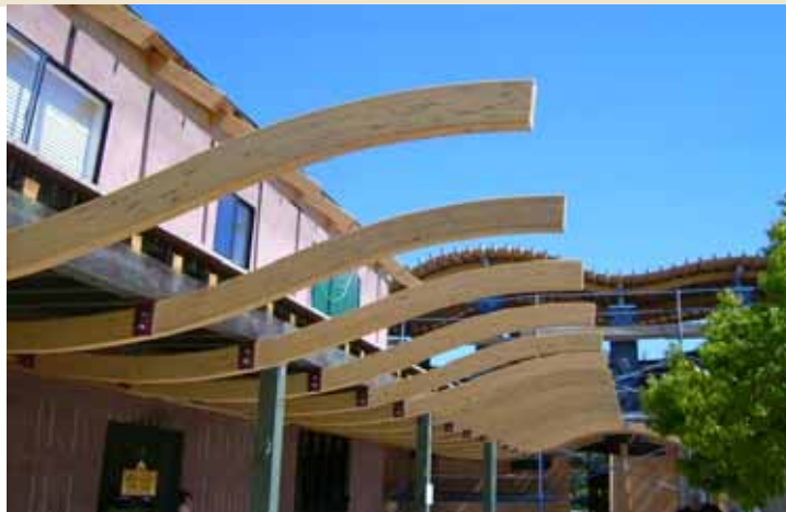
Alaska Yellow Cedar curved Trellis and roof rafters
