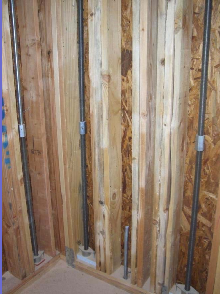
Tie Rods & Compression Studs at Shear Panels
