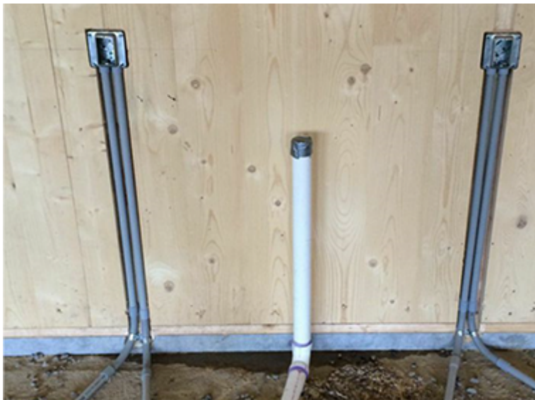
Options for Incorporating MEP in Exposed Mass Timber Structures
