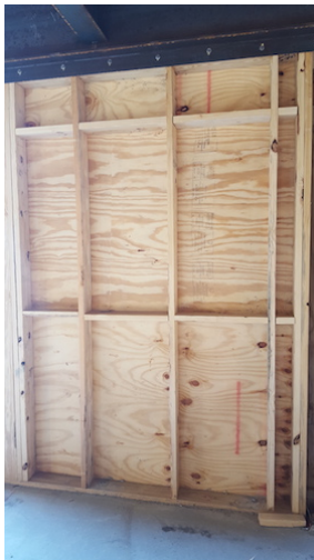
Shear panel edges
