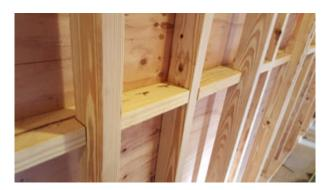
There is no requirement that shear wall panel edge blocking match the depth of the wall studs, nor is there a requirement that it be oriented in the same axis as the wall studs.
