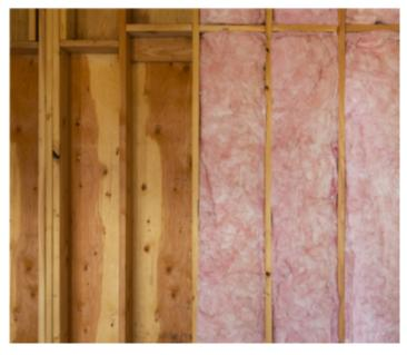
The general rule of thumb when using an assembly that wasn't tested with insulation is that it's ok to add it for walls but an additional ceiling layer of gypsum is required when adding it to floor/roof assemblies. Below are several references to support this.
