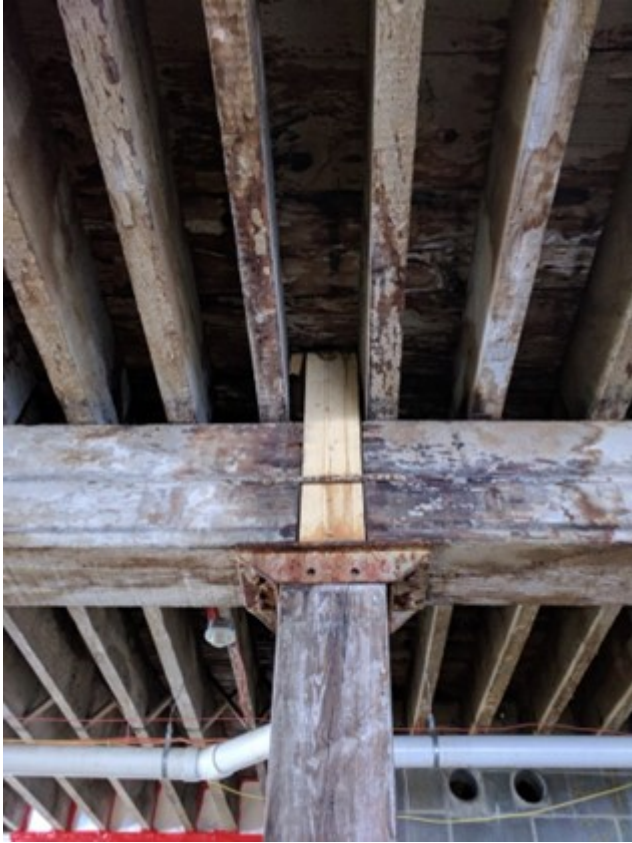
Bottom of new stub glulam column on existing heavy timber column at 69 A Street / Photo McNamara • Salvia
