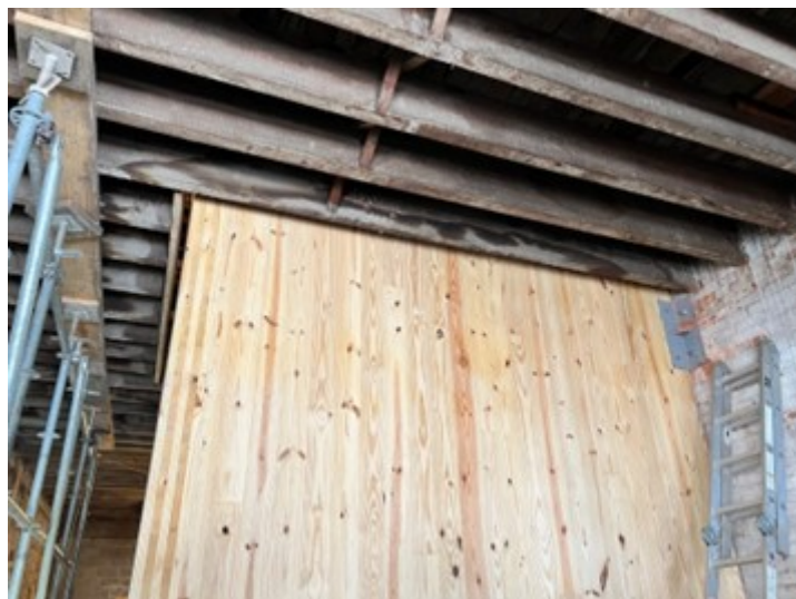
New CLT shaft walls in existing lower three stories of ACME Timber Lofts / Photo WoodWorks
