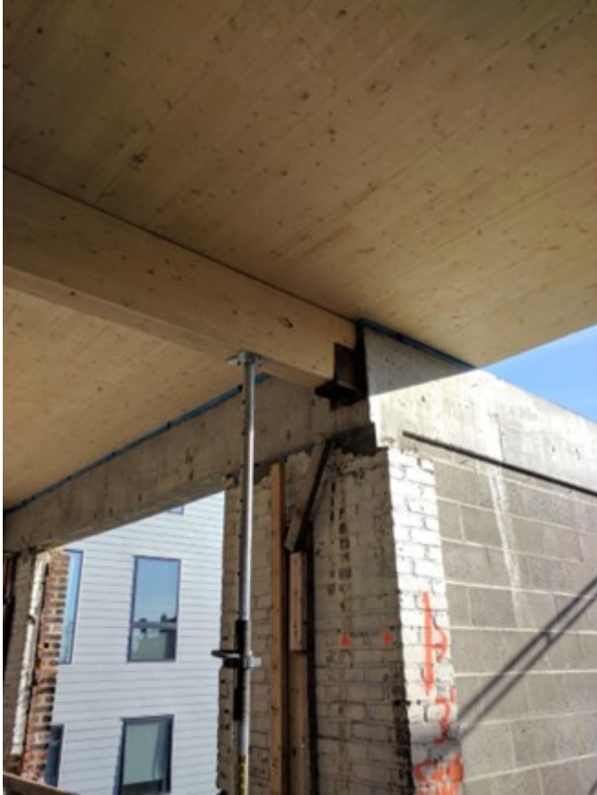
New mass timber framing at new concrete rim beam on top of existing exterior walls at 69 A Street / Photo McNamara • Salvia
