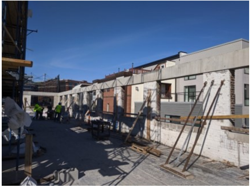
A new concrete rim beam on top of existing brick exterior walls establishes a working surface for a mass timber vertical addition at 69 A Street / Photo McNamara • Salvia
