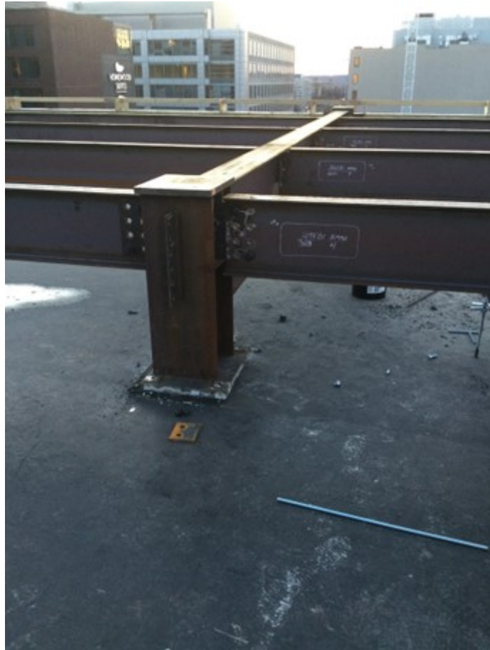
New steel dunnage frame on existing concrete sloping roof / Photo Hickok Cole
