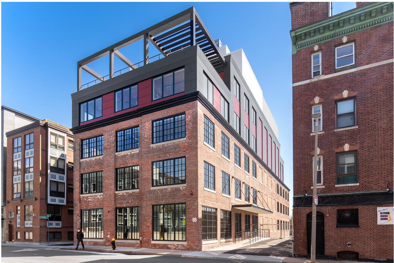
Two-story mass timber vertical addition on existing three-story building at 69 A
