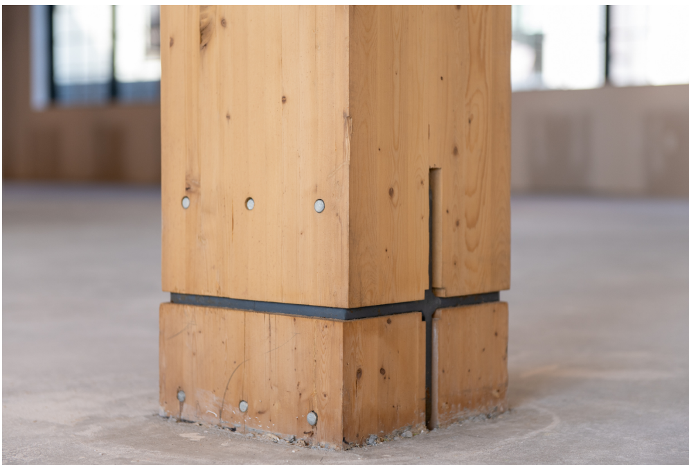
Top of new stub glulam column on existing heavy timber column / Photo Greg Folkins
