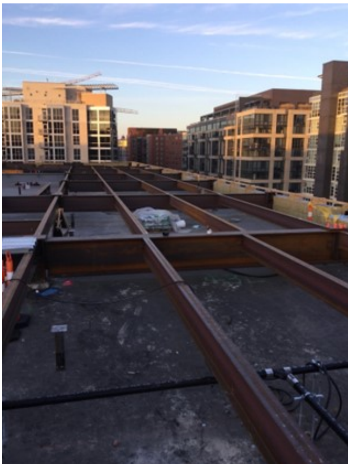
New structural steel framing installed on existing sloped concrete roof slab to establish level working surface for mass timber install at 80 M Street in Washington, DC / Hickok Cole / Arup / Equilibrium / Photo Hickok
