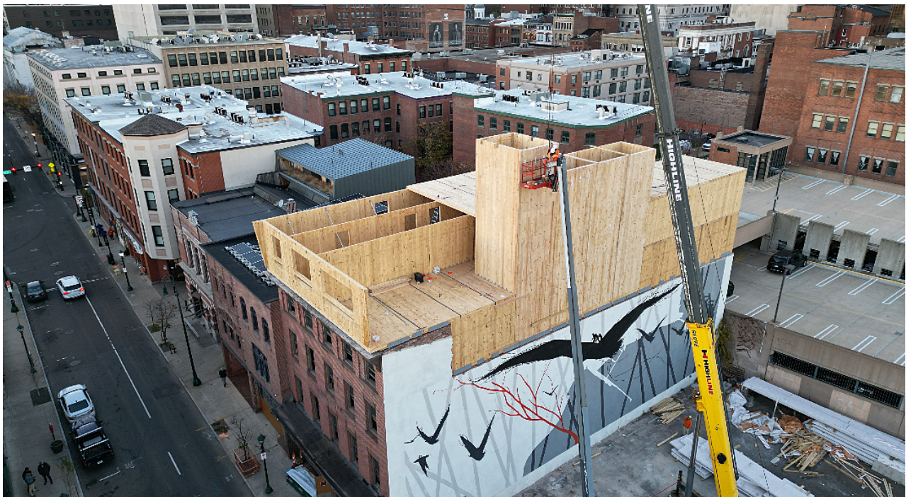
ACME Timber Lofts—a two-story mass timber vertical addition in New Haven, CT / GOA / Odeh Engineers/WSP / Photo GOA
