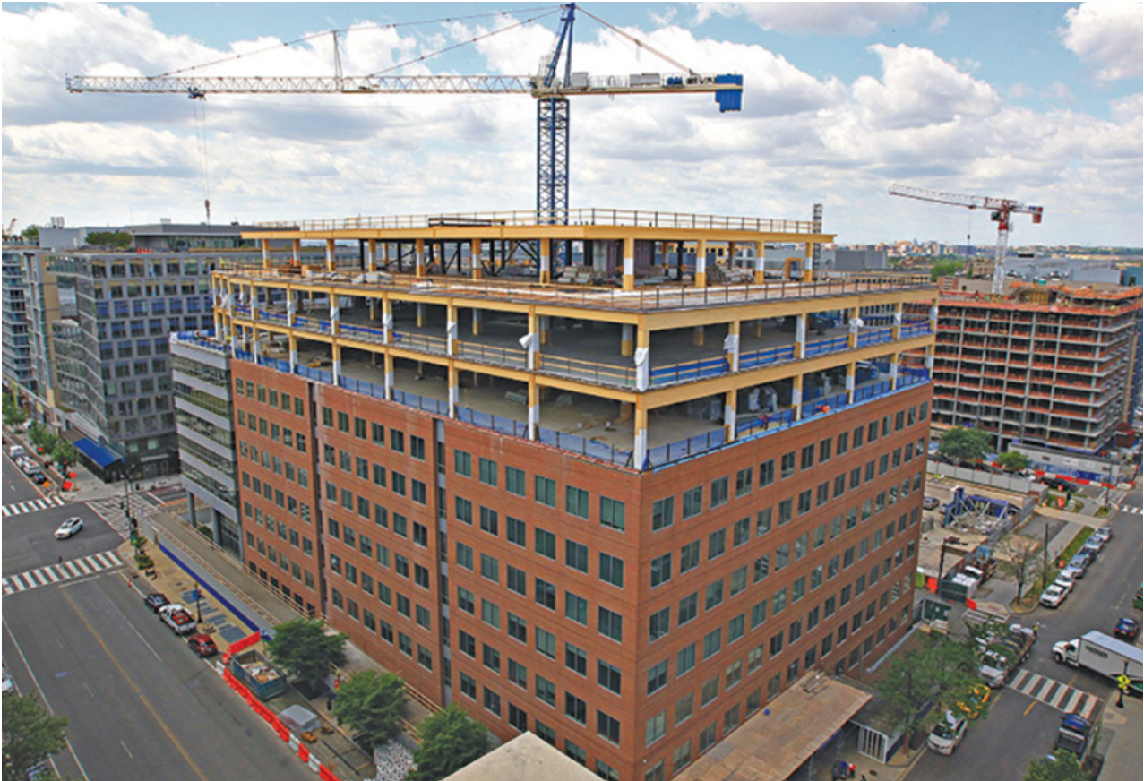
Mass timber addition at 80 M Street in Washington, D.C. / James G. Davis Construction
