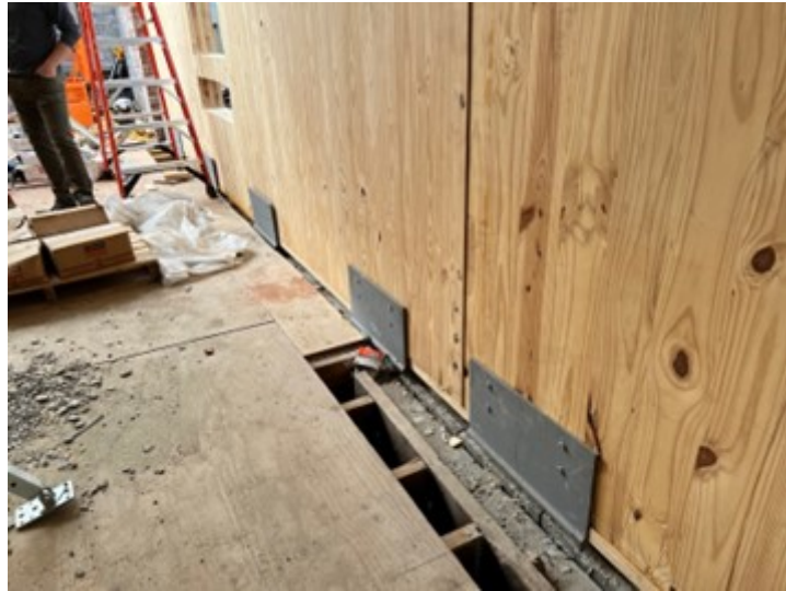
New CLT exterior walls installed on top of existing masonry exterior walls, attached with L-shaped steel plates at ACME Timber Lofts / Photo WoodWorks
