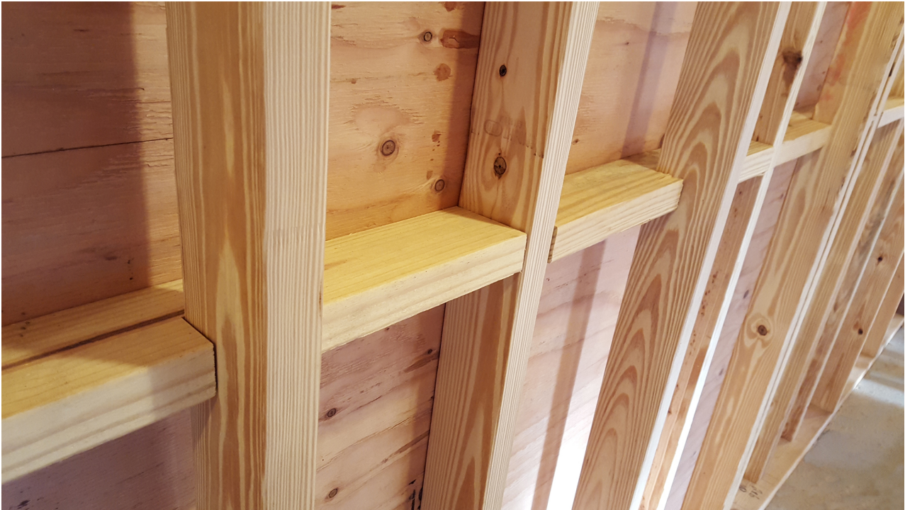
Staggered stud wall with shear wall blocking in contact with both rows of studs, causing sound transfer touch point / Photo WoodWorks
