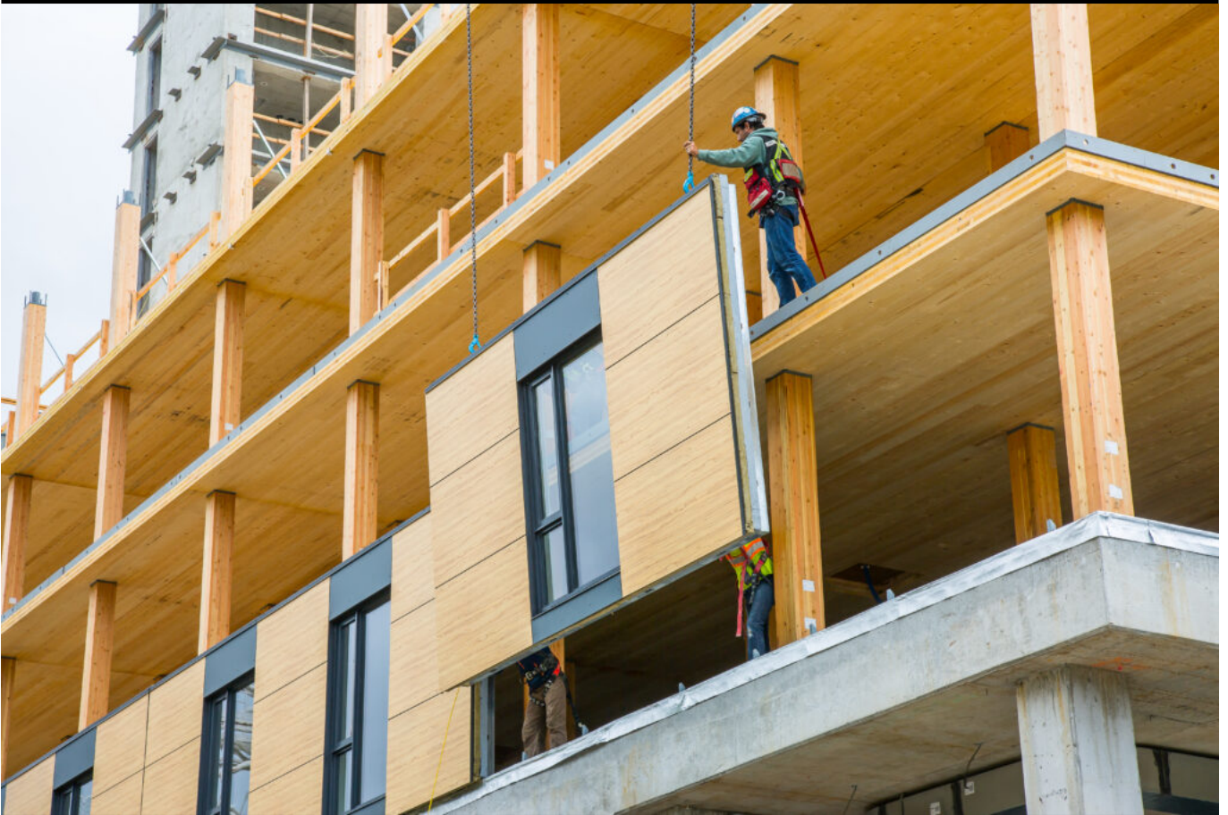
Mass timber building with prefabricated, noncombustible exterior curtain walls Brock Commons Tallwood House, Vancouver, BC Acton Ostry Architects | Photo: naturallywood.com
