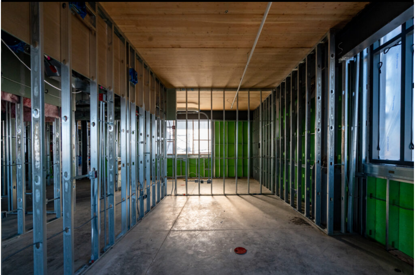
Mass timber building with light-gauge steel stud exterior walls Beaverton Public Safety Center, Beaverton, OR
