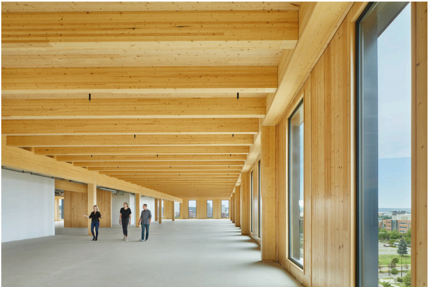
Mass timber building with prefabricated, combustible exterior curtain walls Catalyst, Spokane, WA
