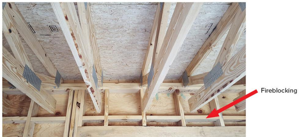
**FIGURE 2:** Fireblocking in wall cavity at intersection with floor
