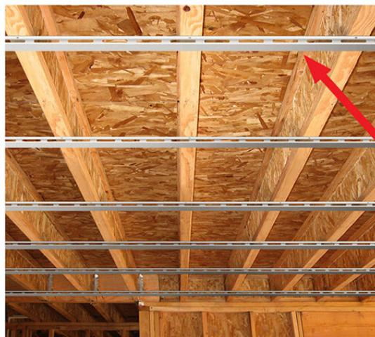
Composite wood joist construction with ceiling channels attached, prior to installation of batt insulation and compartmentalization materials
