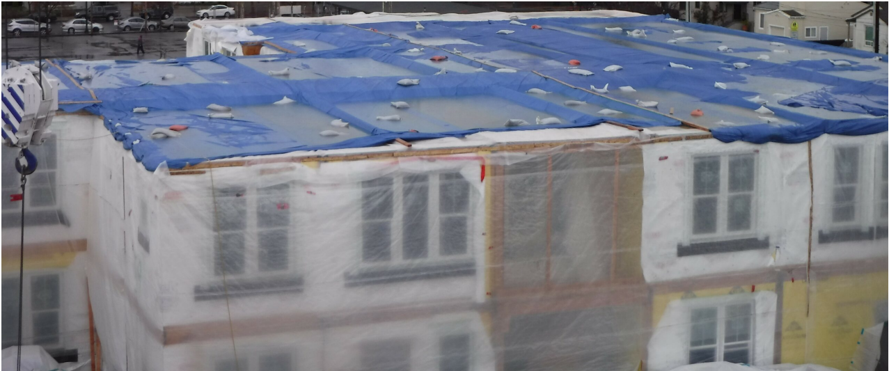
Figure 6 – Pooled water over tarps installed at intermediate module roofs
