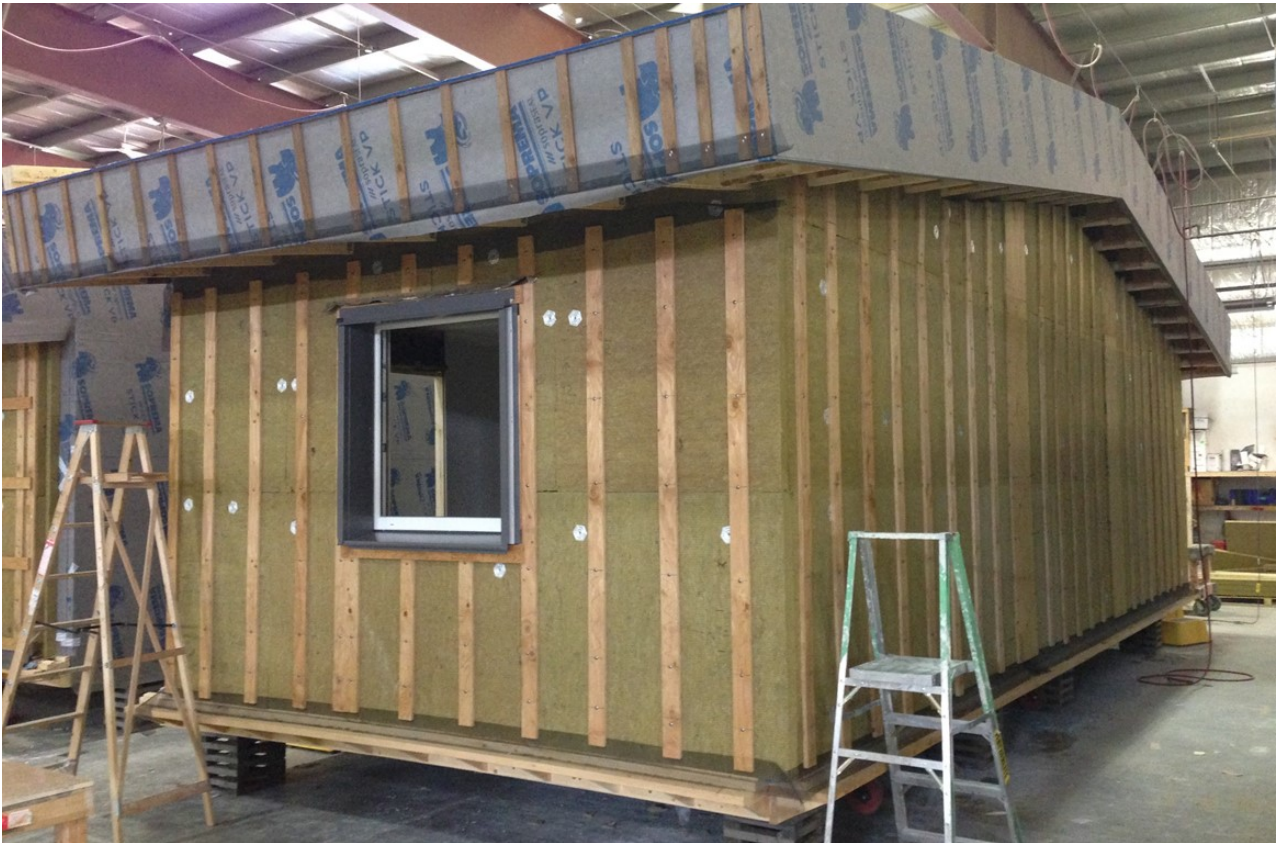
Figure 7 – Exterior insulation installed on a module in the factory
