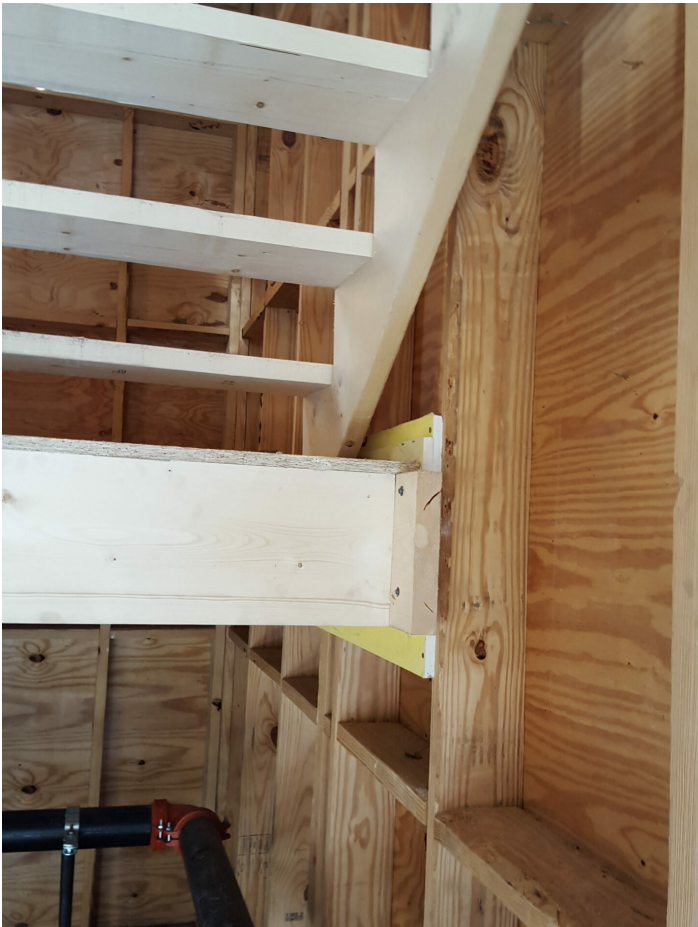
Stair landing framing attached to shaft wall through two layers of gypsum prior to landing beam hanger installation
