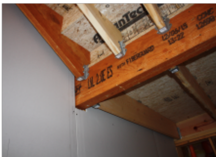
Stair landing beam shaft wall structural penetration prior to firestop system installation
