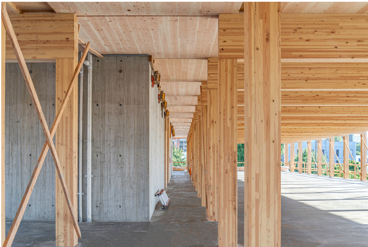
Two-way CLT is used for a beamless zone adjacent to the core at District Office in Portland, OR / Photo Hacker
