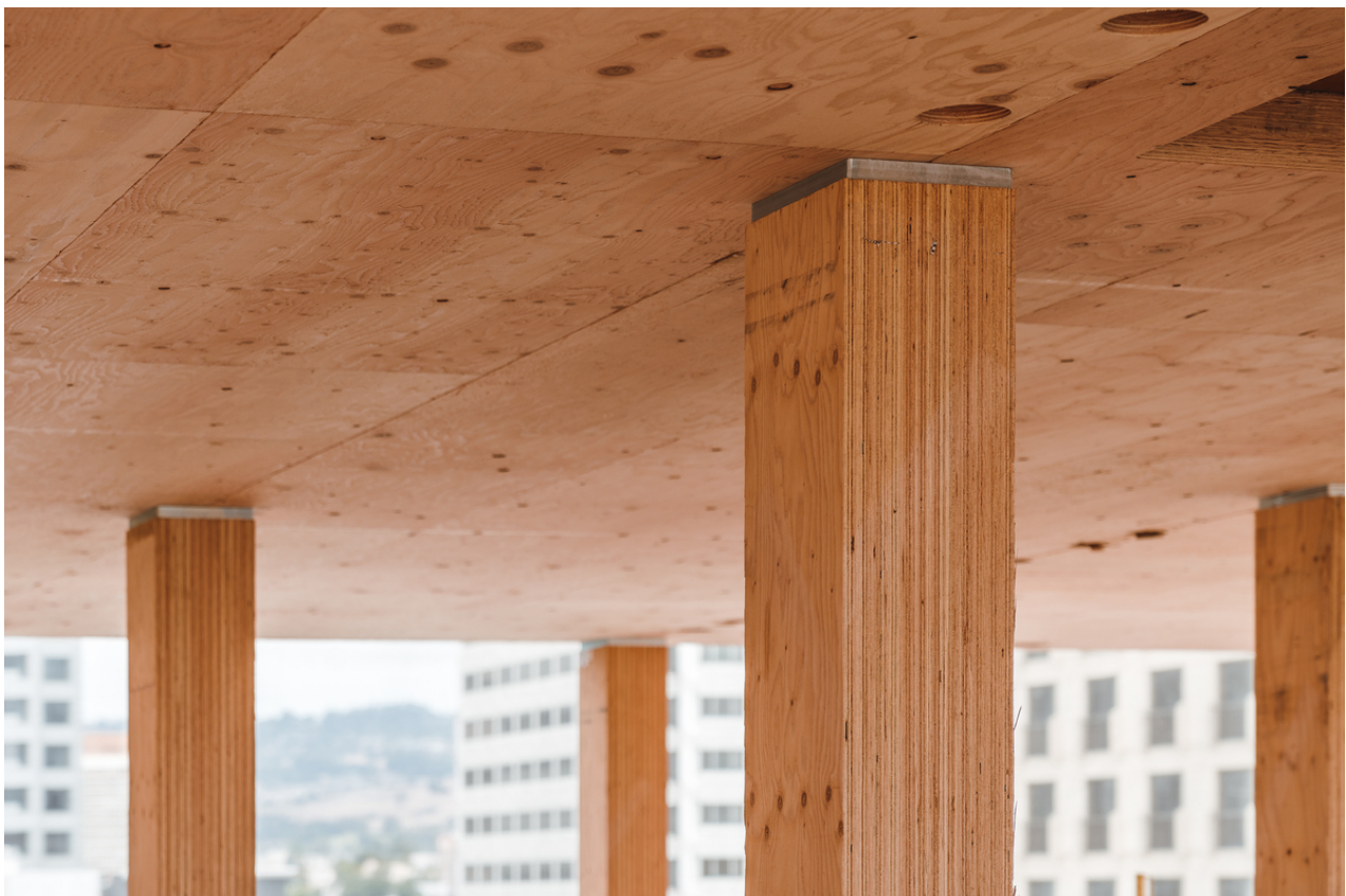
CLT panels made from SCL laminations span two ways at 1510 Webster in Oakland, CA / Photo WoodWorks
