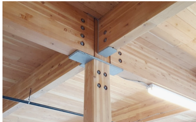
Unprotected exposed connections
