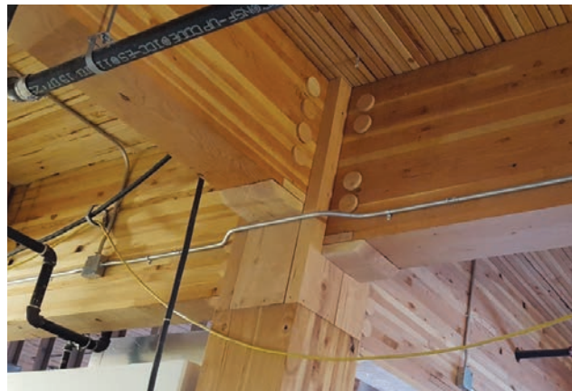
Exposed connections protected with wood coverings
