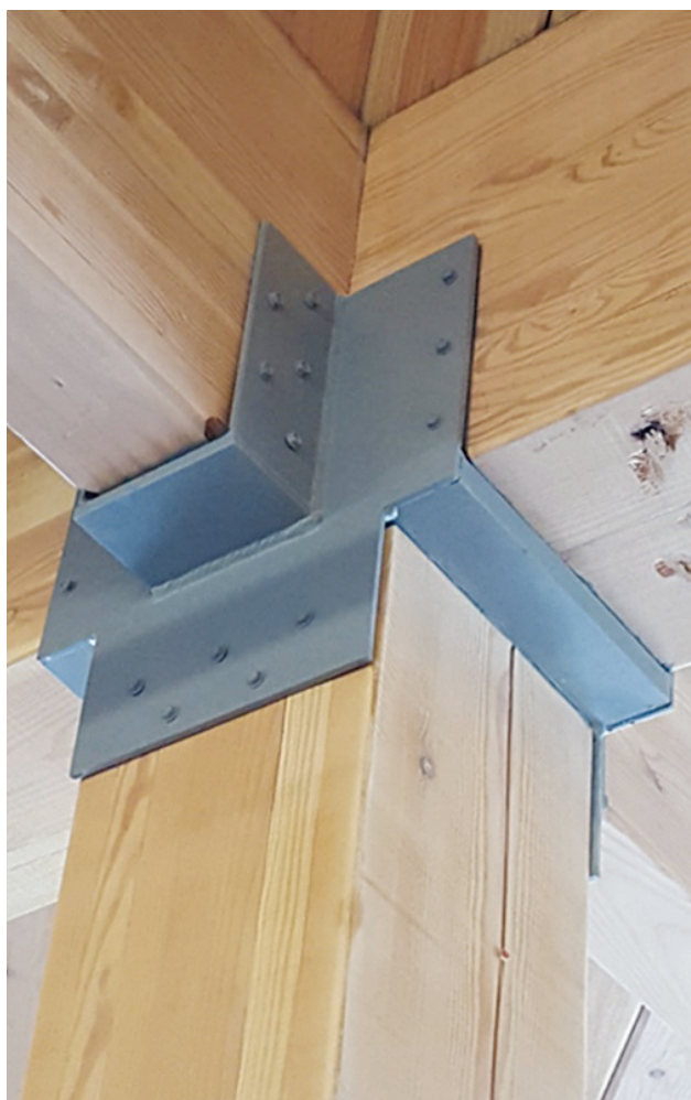
Connection protected and approved using other means acceptable to the jurisdiction
