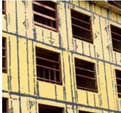
Sealed Gypsum Sheathing – Sealant Filler at Joints
