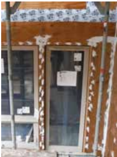
Sealed Plywood Sheathing – Sealant & Membrane at Joints
