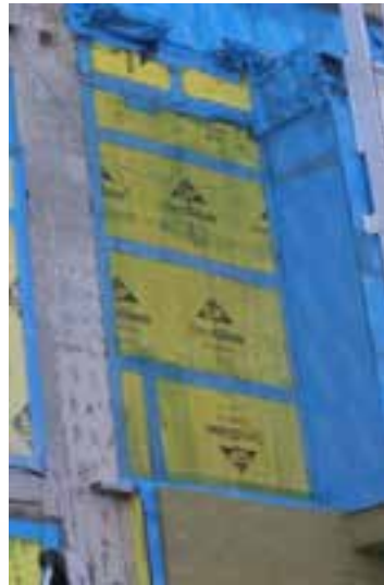
Sealed Sheathing – Membrane at Joints
