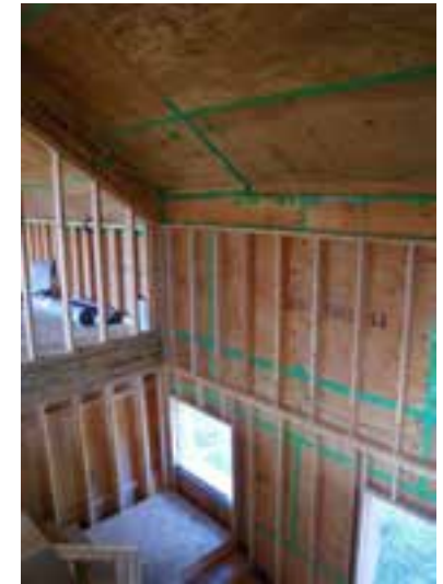
Plywood sheathing with taped joints (good tape)
