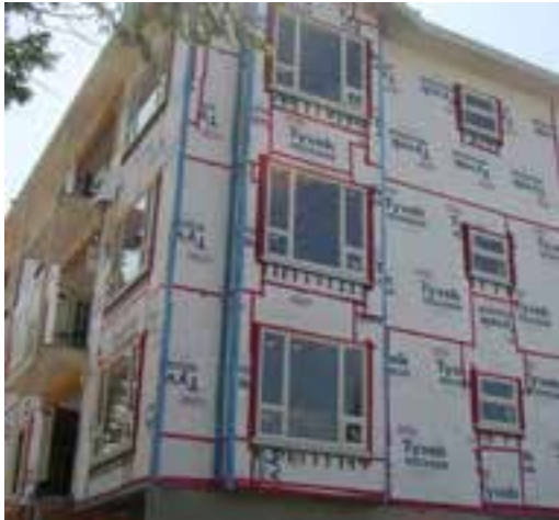
Loose Sheet Applied Membrane – Taped Joints & Strapping
