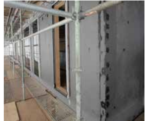
Liquid Applied – Silicone sealants and silicone membrane at Joints
