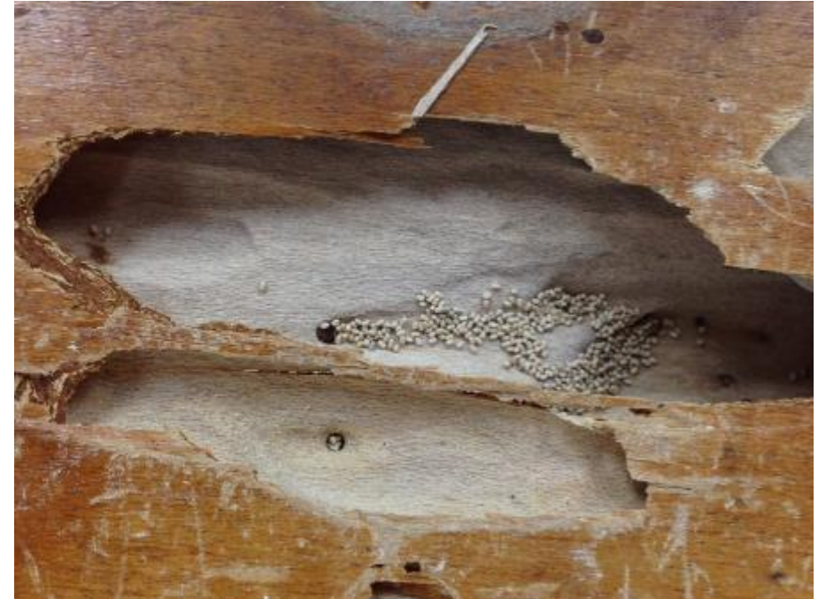
EVIDENCE AND DAMAGE
