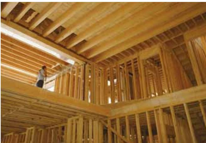
Hundreds of structural elements and thousands of nail connections provide alternate load paths.
