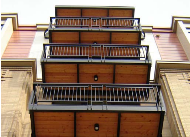
Heavy timber decking used on balcony
