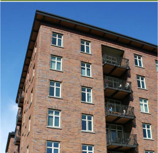
Balcony elements inset to exterior walls
