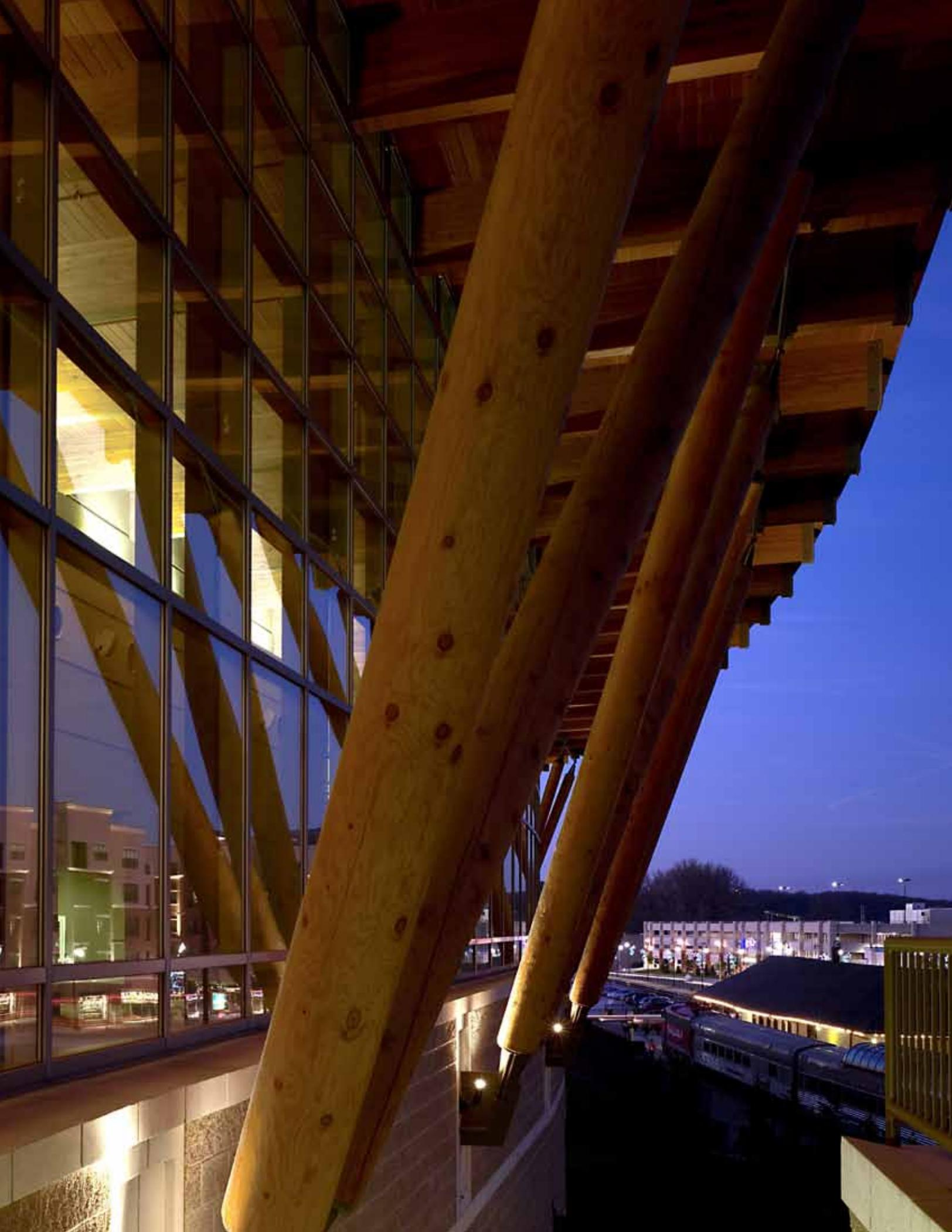
**H**eavy timber construction—used for hundreds of years around the world—successfully combines the beauty of exposed wood with the strength and fire resistance of heavy timber.
