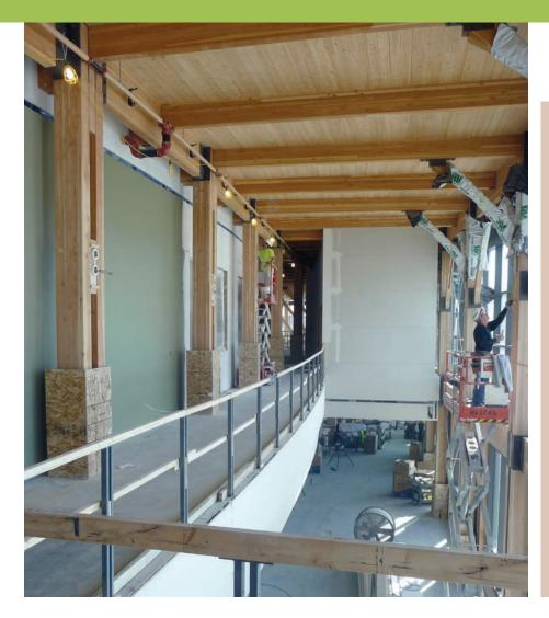
had specific requirements. The code reviewer interpreted the wood portion of the building as being better or equal to the GMP structure in terms of fire resistance. So the whole structure is actually classified as a Type II-B steel frame structure. We just had to show that The Crossroads timber portion had equivalent performance, which we did."
