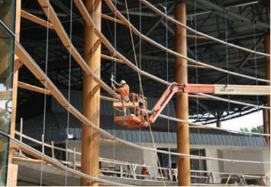
Once the columns were installed, crews stretched pre-tensioned cables along the perimeter of the façade and then locked the PSL muntins and support arms into place. When they hung the glass off the cables, everything settled to its proper position.
