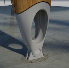
Weighing about 10,000 pounds each, the PSL columns were shaped to an elliptical cross-section and fit into delicate-looking but structurally efficient ductile iron castings designed to bring the enormous 400,000-pound roof loads down to a single pin.
